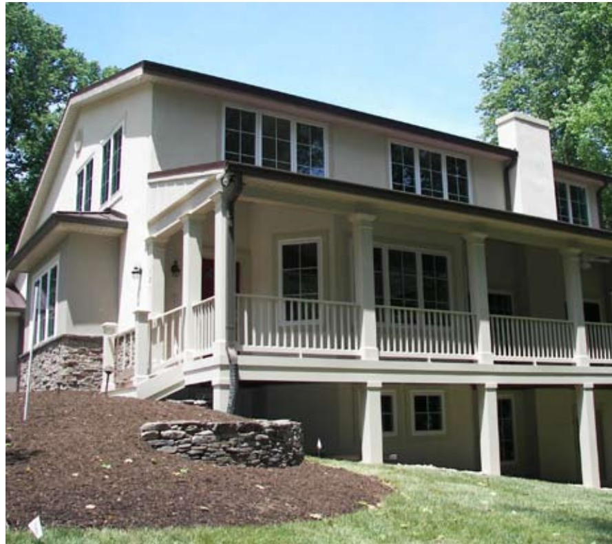
Steel and cement home under construction, in the framing stage (top) and with stucco finish and stone accent (above).
